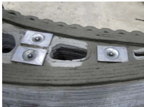
3. Functional voids and reinforcement close-up
